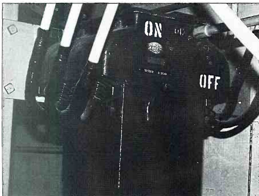
This ac switch was found in the basement of a transmitter building. Note the oil-fill plug on the front panel.
